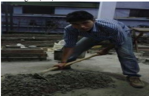
Figure(2.1). Mixing of concrete material
